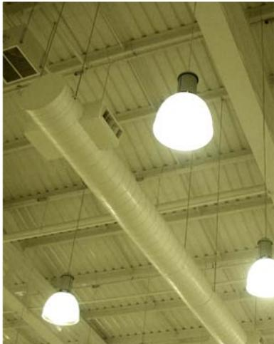
The recovered 'free' heat from the refrigeration system was used to meet all of Aldi's heating needs.
